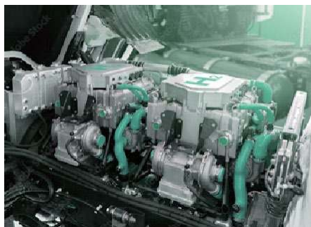
Fuel Cell Discharge Testing
