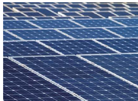
Solar Array Load Testing
